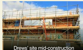
Drows' site mid-construction
