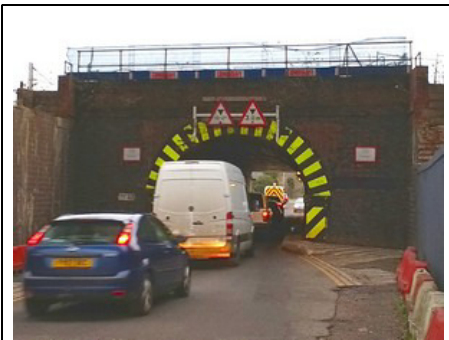
BOTTLENECK: Cow Lane railway bridge
