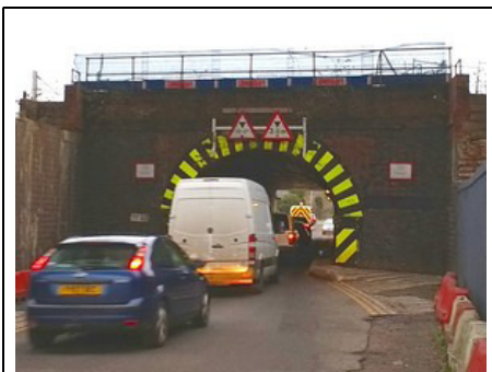
BOTTLENECK: Cow Lane railway bridge
